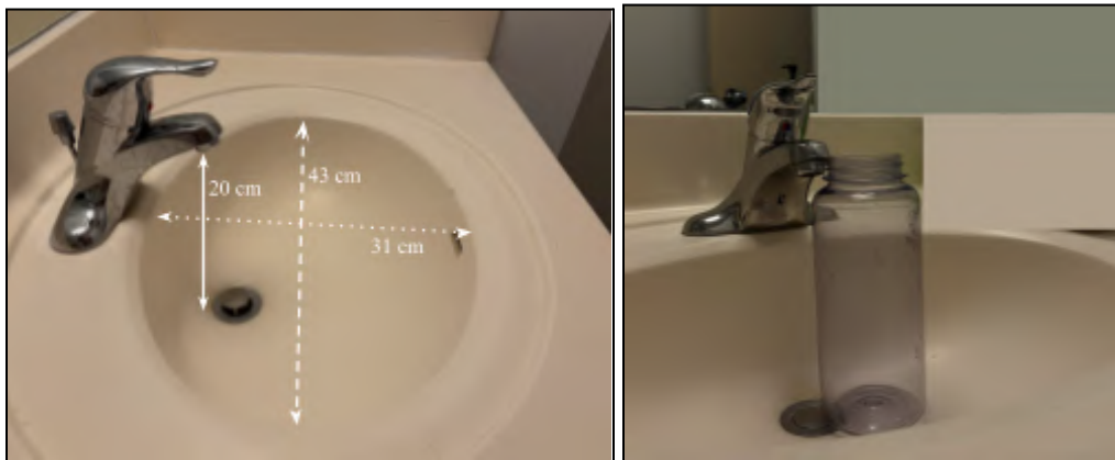
Figure 1. Dimensions of sink and tap configuration (left) and height comparison of faucet and bottle (right).
